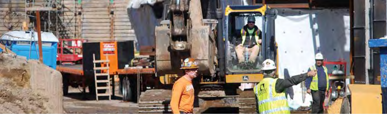
Baystate Medical Center construction project, Springfield, MA
